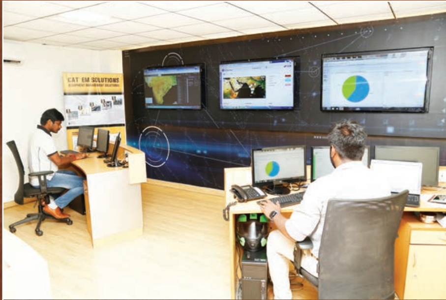
EM Solutions Control Room, Chennai
